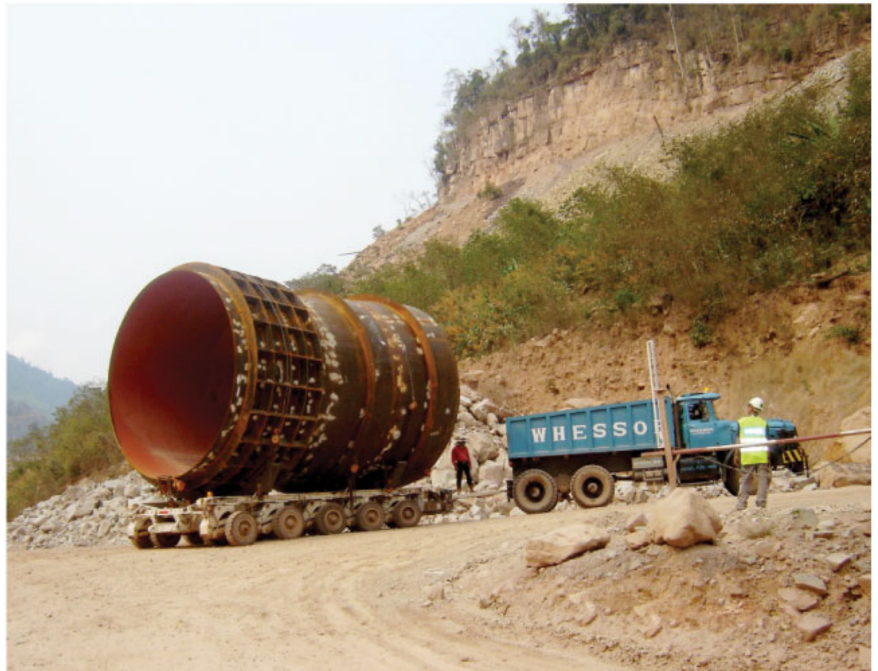
EPC Contract for the design, supply, fabrication and installation of 3,500 tonnes of steel lining and manifold.
